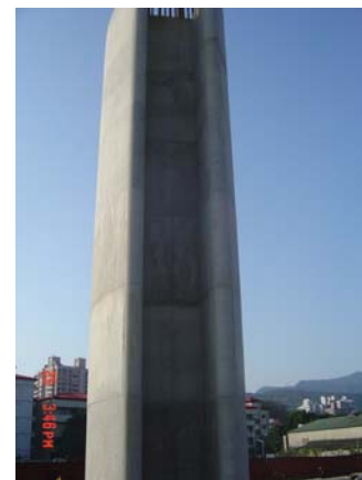
Picture 20 SCC on columns of BaLi-WuGu Freeway
