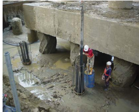
Picture 4 Cast-in-place pile
