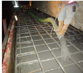
Picture 17 Placing SCC
