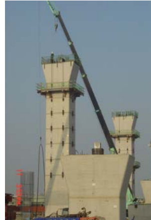
Picture 19 Erected of column
