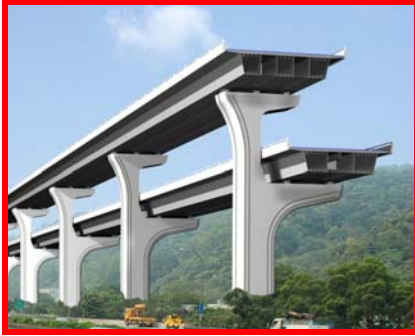
Figure 21 Double deck Bridge
