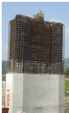
Picture 1 Dense Rebars at column Picture 2 Labor cost and noise of vibration
