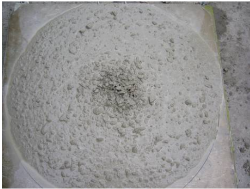
Picture 28 SCC segregation
