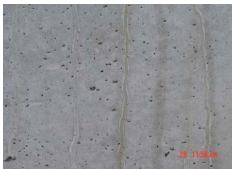
Picture 30 SCC surface easy to create air void due to no vibration
