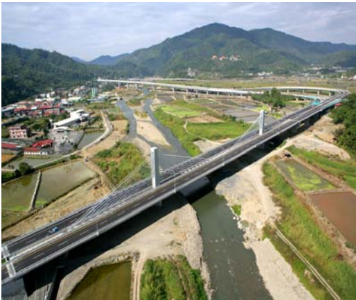
Picture 8 Ai-Lan Bridge
