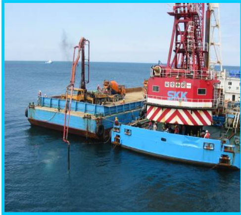
Picture 3 Concreting under water
