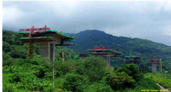
Picture 15 V-Shape Column
