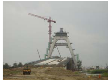
Figure 6 Da-Pan Bridge applied SCC on pylon and piers
