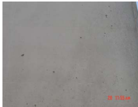
Picture 30 SCC surface easy to create air void due to no vibration
