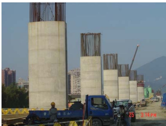
Picture 20 SCC on columns of BaLi-WuGu Freeway
