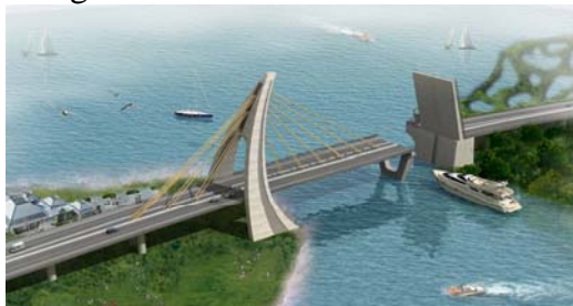
Figure 6 Da-Pan Bridge applied SCC on pylon and piers
