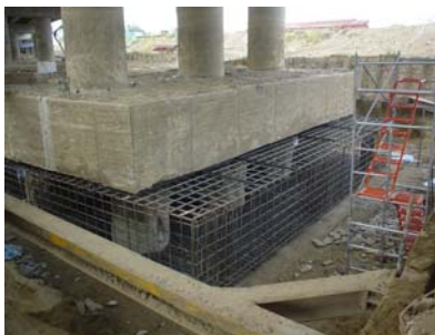
Picture 16 place reinforcement
