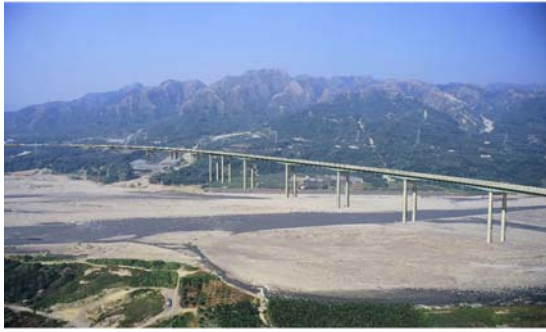
Picture 10 Kao-Sen Interchange Viaduct
